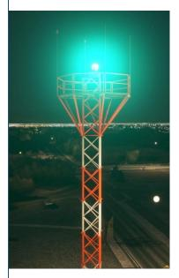
Airfield lighting will generally be one of two extremes. The airport may come to life after dark with an array of runway and approach lighting systems, or fade away into the darkness and be impossible to see. Airfield lighting in the USA usually includes an airfield beacon, which rotates on top of a tall mast and is seen as a flashing green and white light, making picking out an airfield surrounded by built up areas easier.
