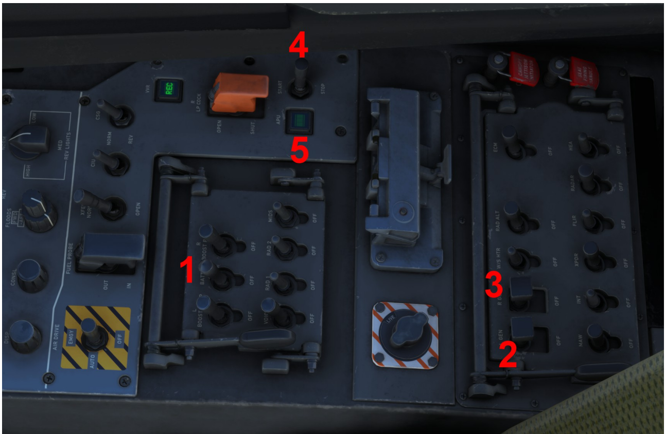
ELECTRICAL POWER SUPPLY SYSTEM CONTROLS (right consoles)
